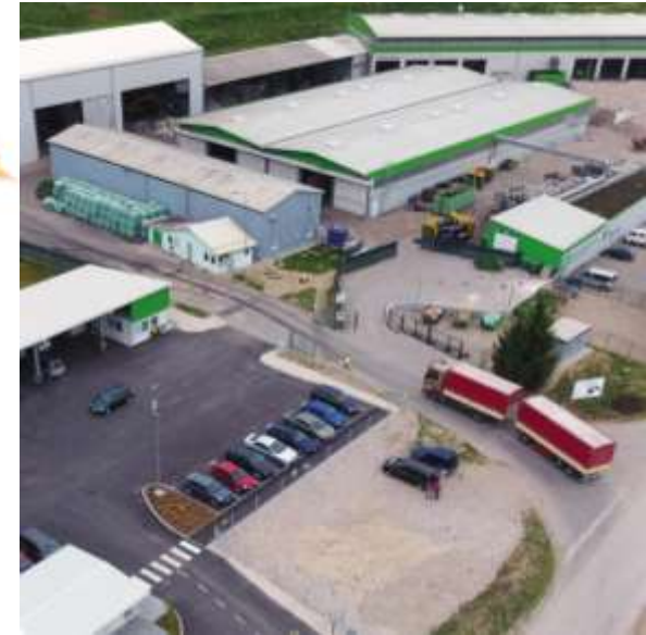
(c) Waste recycling centre Krško
