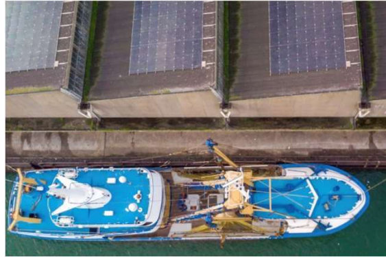
Port of the Hague has installed photovoltaic panels in its facilities (Getty images)
