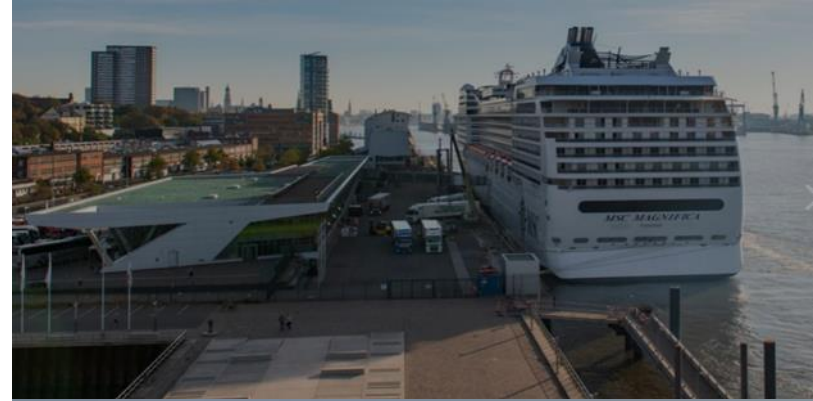
Figure 1: Hamburg port on shore power supply project
